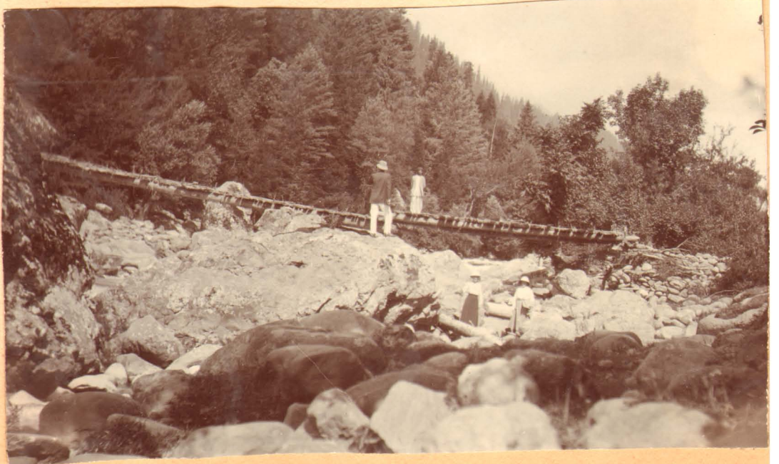
W. Linder stream & bridge
